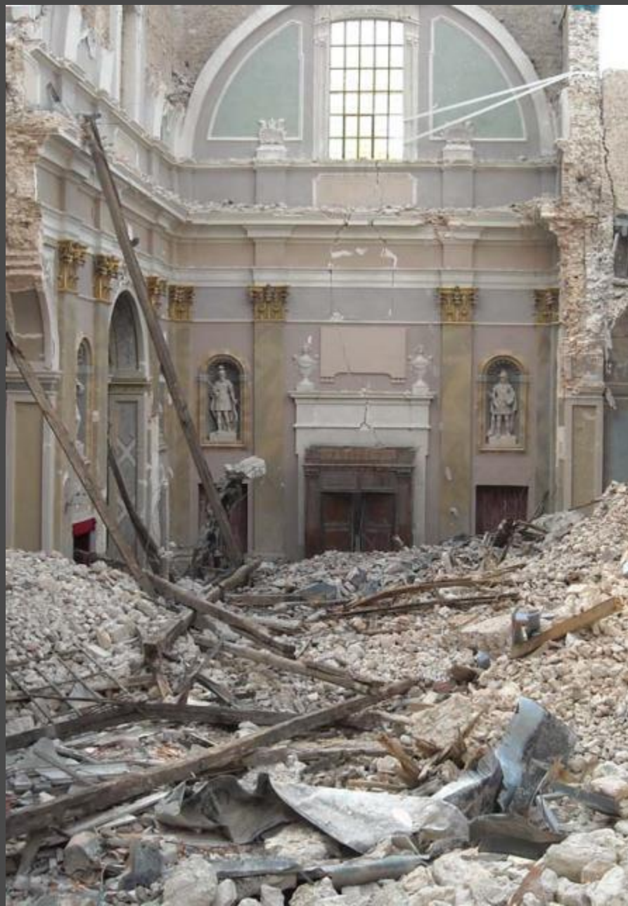
S. Maria Paganica, after collapse and proposal for reconstruction
