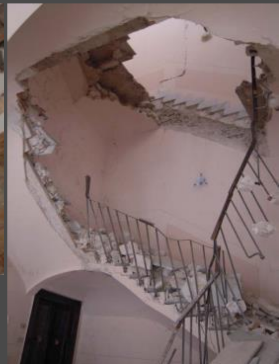
Staircase with damaged stairs in a building in via Roma
